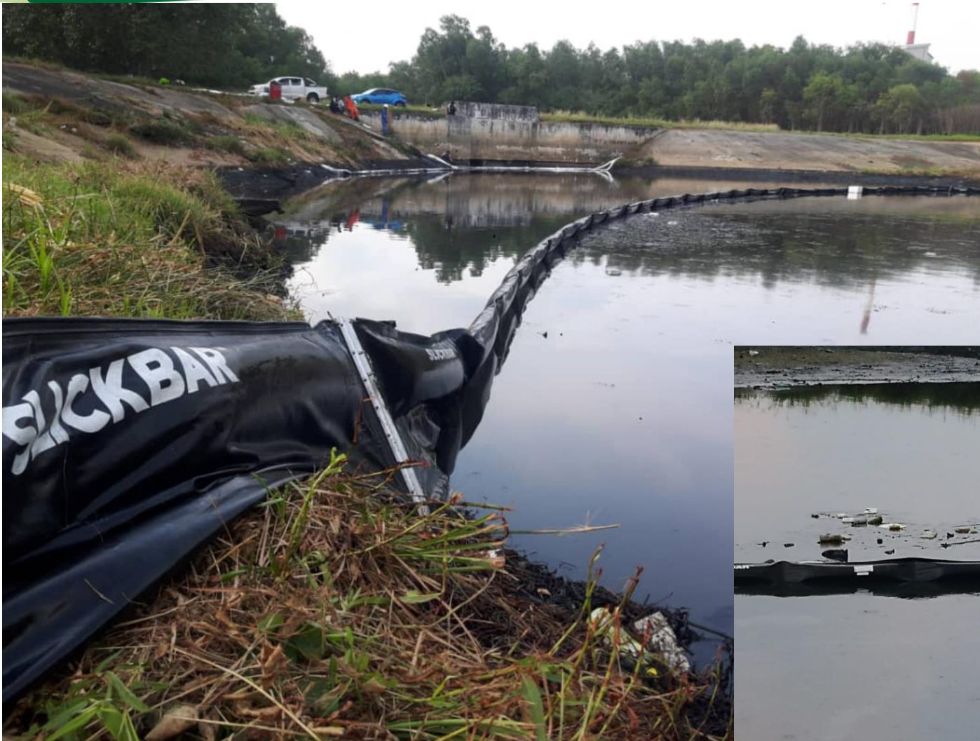
16 Apr 19: Deployment of solid floatation boom as 2nd line of defense to contain further oil
